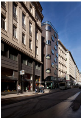
© BWM Designers & Architects
