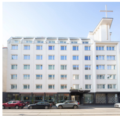
© BWM Designers & Architects
