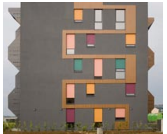
↑ End facade with bedroom windows.
