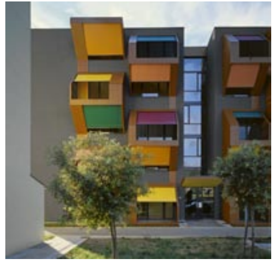
↑ View from street of glazed entrance and staircase.
