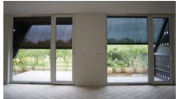
↑ View through the full-height windows and loggia.
