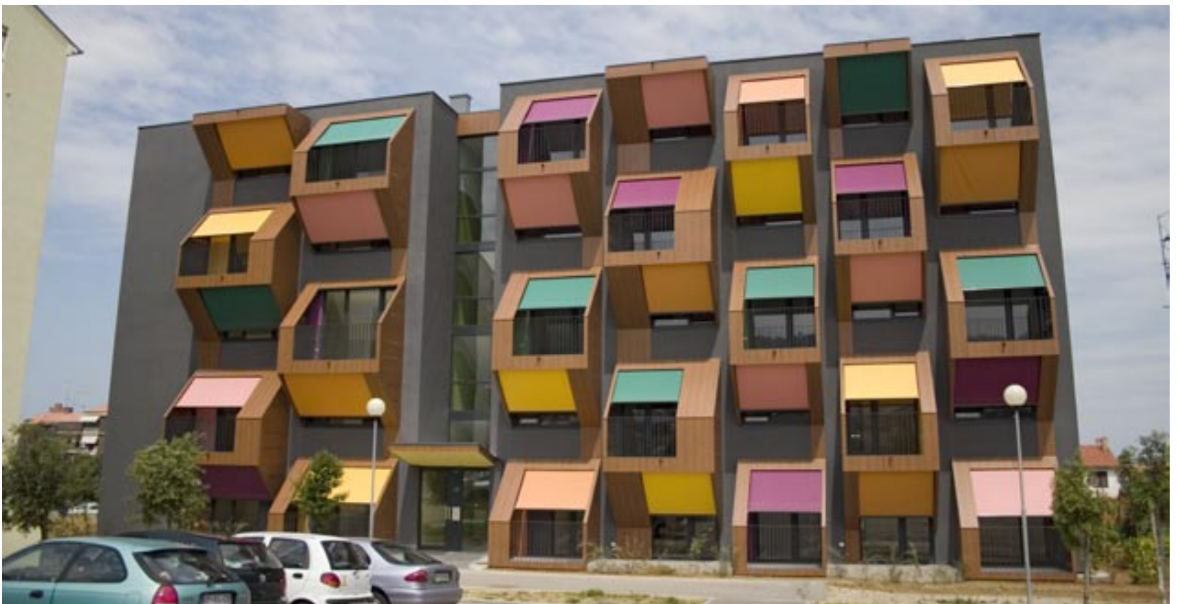
↓ Apartment block by Ofis in Izola.
